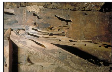
Figure 7. Wood damaged by mature carpenter ants.
