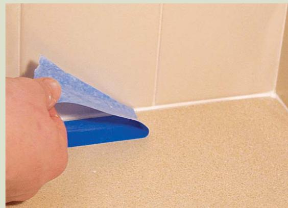
wise, **you can use a sponge, a spoon, the corner of an old credit card,** or any other disposable item that fits the shape of the joint. When tooling silicones or solvent-base sealants, a little soapy water will keep caulk from sticking to the tool. **Remove the tape but protect the area until the caulk has cured.**
