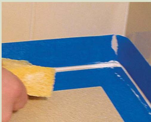
Tooling the caulk after it is applied is not necessary. But if you are not confident that you got enough caulk into the joint or if you want your work to have a smoother finished look, **tool the bead immediately after application.**
