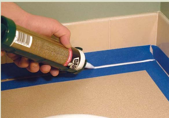
gun as long as you get enough caulk into the joint for it to bond to both substrates. **Tape the sides of the joint to protect surrounding areas from residue,** and know how your caulking gun operates so that you can release the pressure when you stop, to avoid having any extra caulk spill out of the tube.
